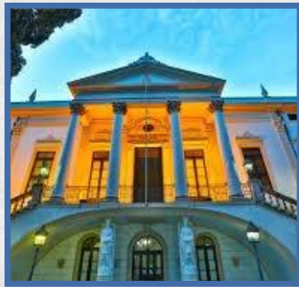
Hospital Santa Izabel
